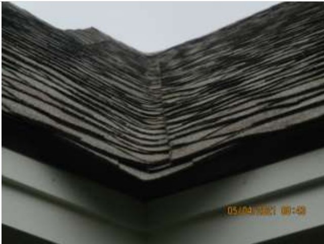
ROOF VALLEY - EAST REAR
