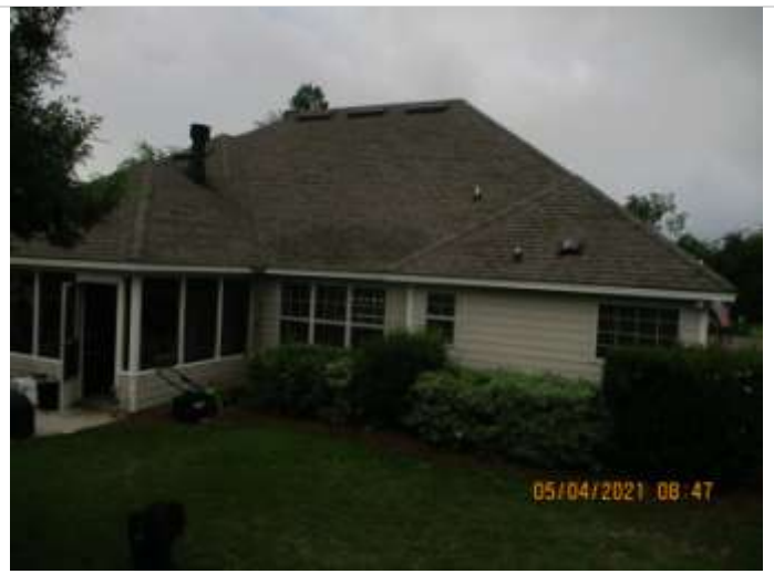
REAR ROOF WITH PENETRATIONS
