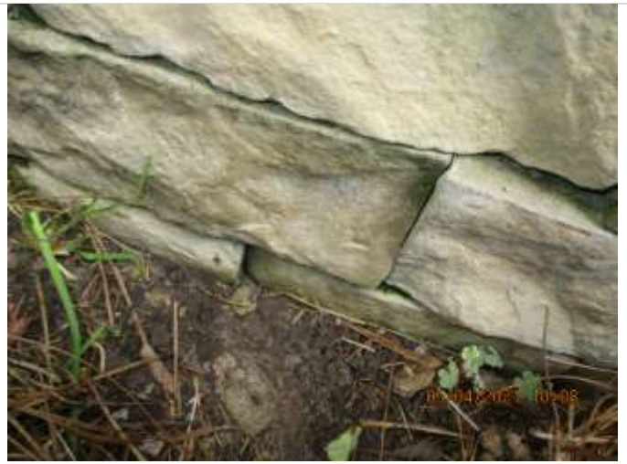
Monitor decor brick for fit and strength
