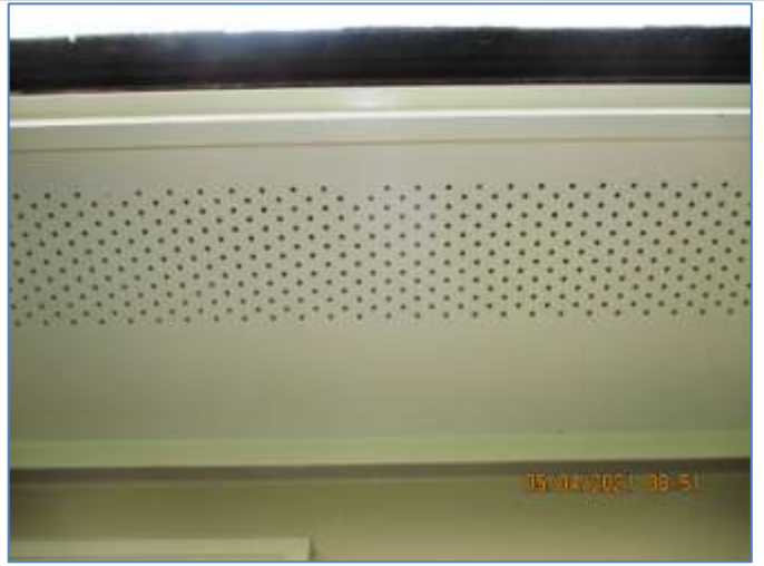
All soffits & fascia were in very good condition.
