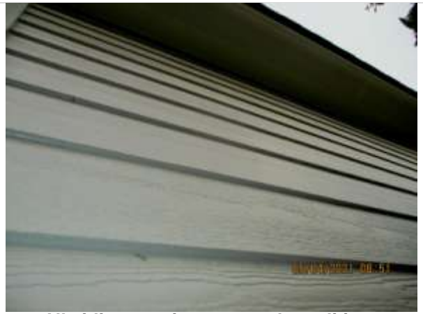
All siding was in very good condition.
