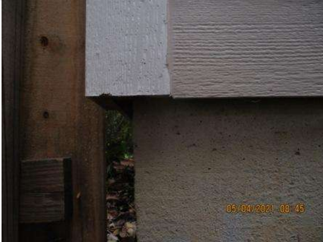
Proper view of exposed foundation : at least 8 inches above grade level
