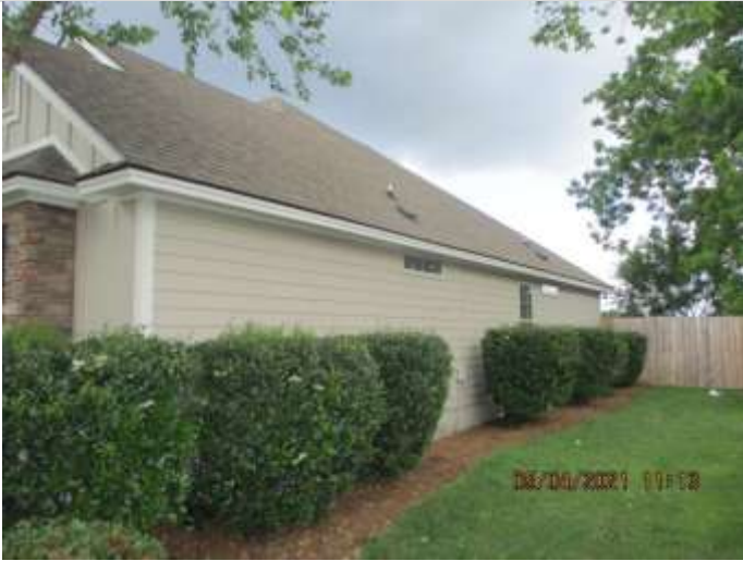
EAST SIDE - GOOD CONDITION
