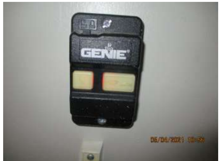
GARAGE DOOR OPENER NEAR HALL DOOR
