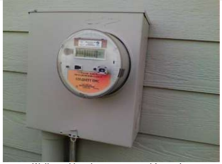
Walls and box have new matching paint
