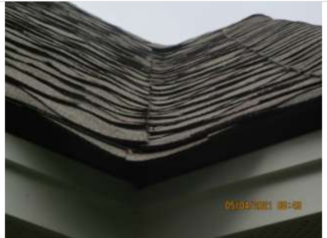
ROOF VALLEY - WEST REAR
