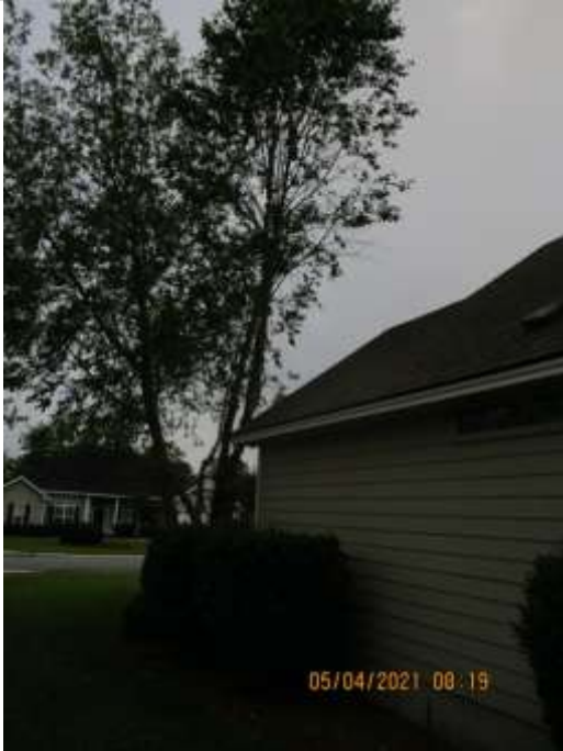
EAST SIDE ROOF VIEW
