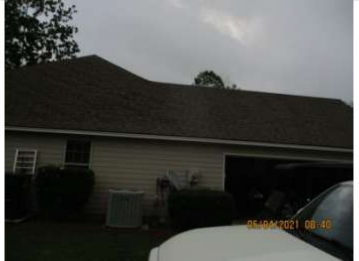
WEST SIDE ROOF VIEW
