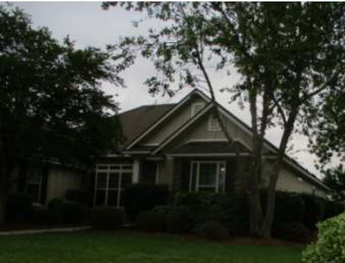
FRONT OF HOUSE - EAST END
