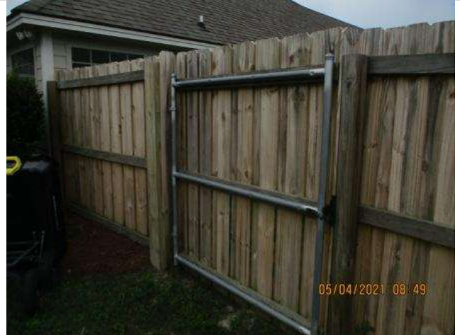
Fence & Gate in Good Condition
