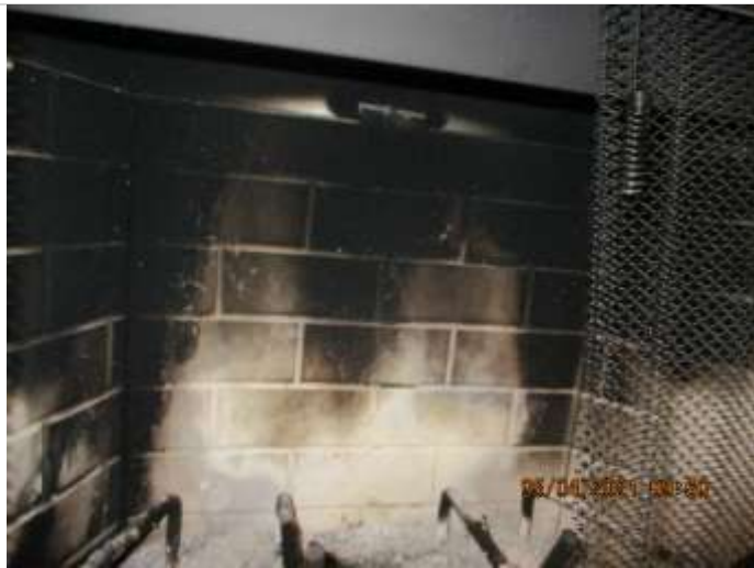
Fire Box Walls
