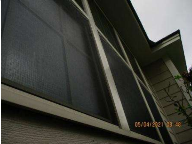
Windows / Screens appeared in good condition
