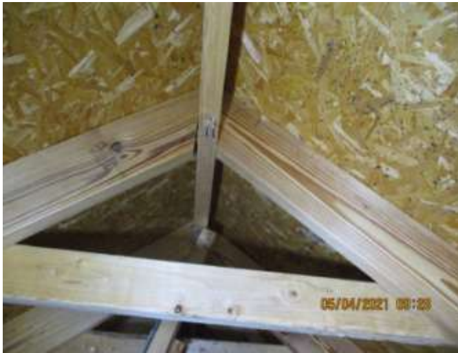
FRAMING APPEARED IN GOOD CONDITION
