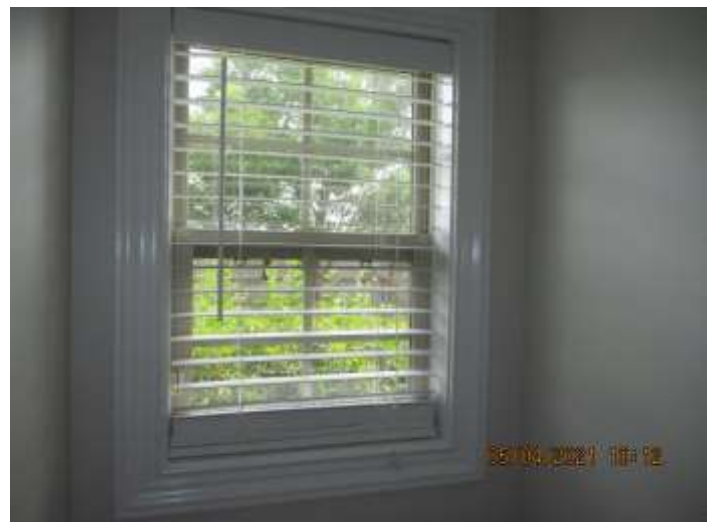
ALL WINDOWS APPEARED IN GOOD CONDITION
