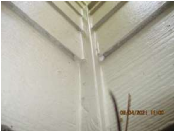
Good Exterior Sealing
